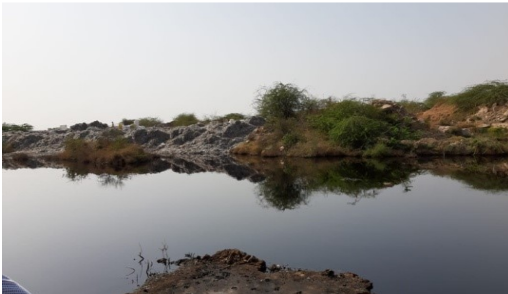
Plate-5Alllegal wastewater & tar in Natural drain/depression leading to River Mahanadi, Ranekpar ,Morbi
